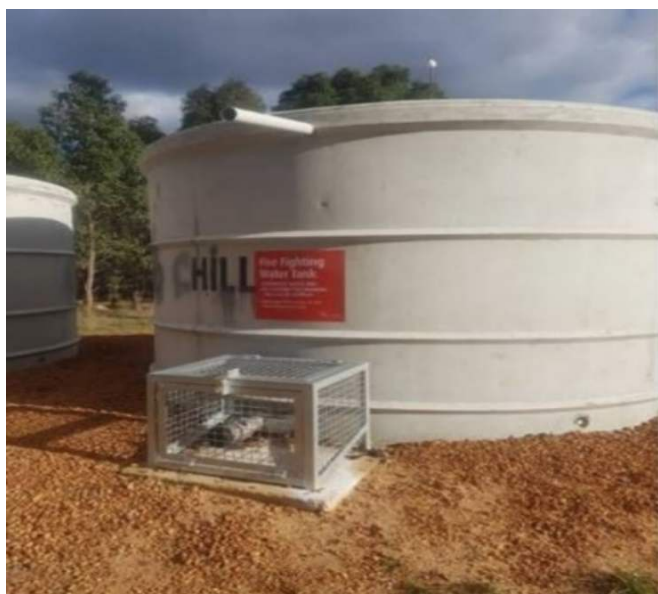
Example Strategic 47,000 Litre Concrete Tank & Protected Fittings
