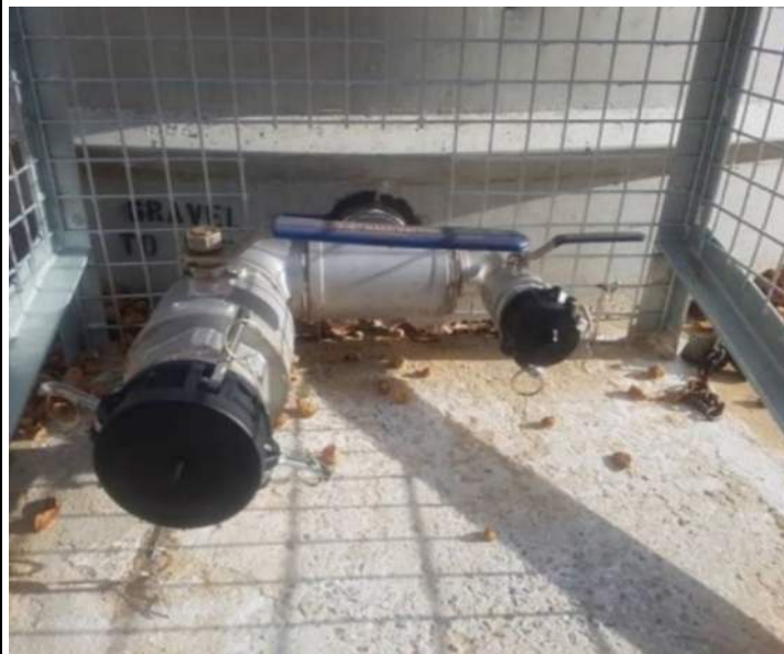
Example Strategic 47,000 Litre Concrete Tank & Protected Fittings
