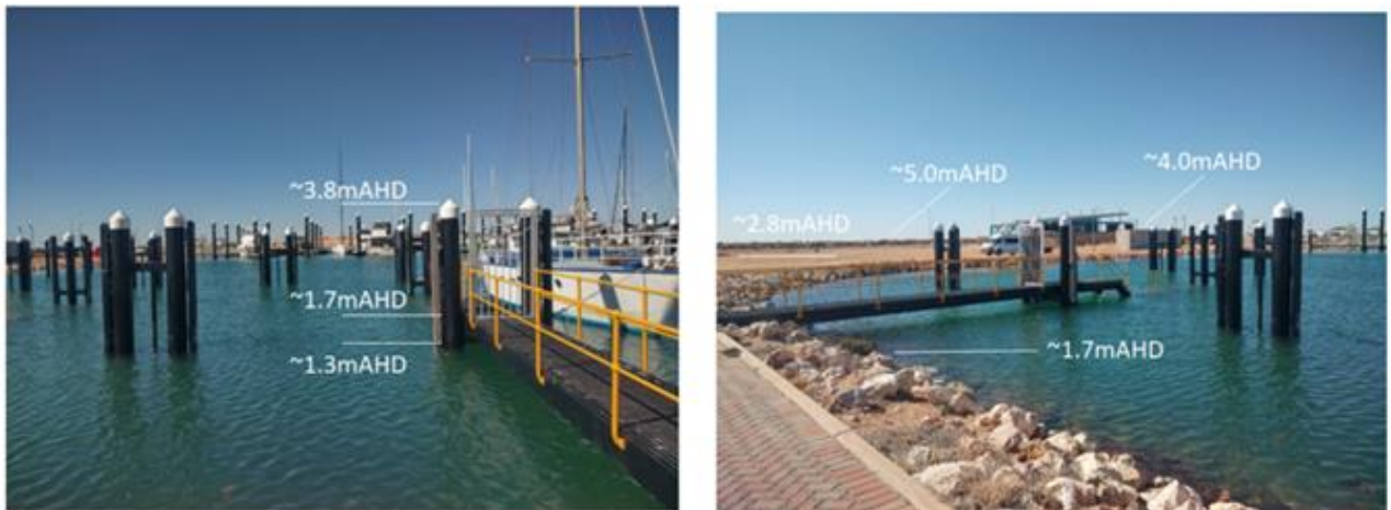
Figure 6-25: Harbour Infrastructure Levels, MU3
