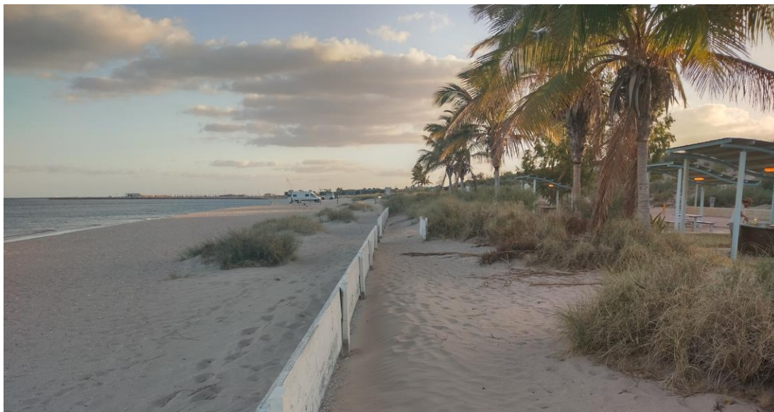
Figure 4-1: Town Beach foreshore assets located within the erosion hazard zone.
