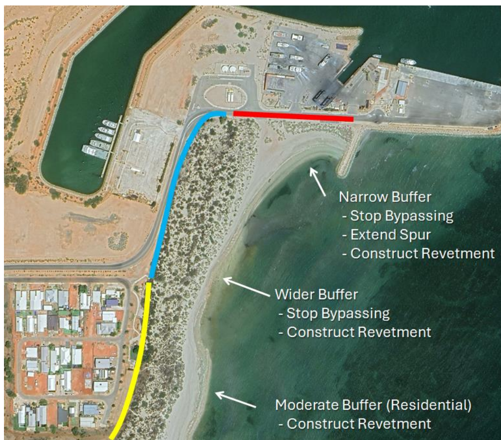
Figure 6-29: Segments for Neale Cove Erosion Management
