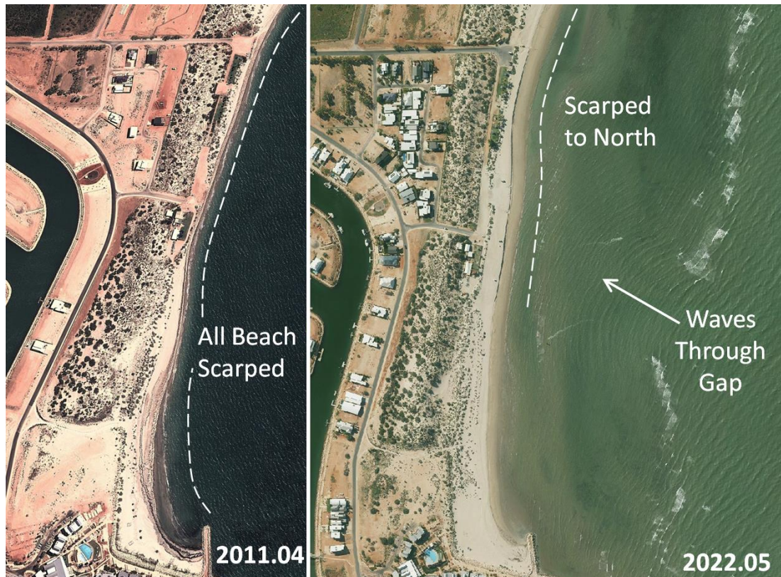
Figure 2-6: Observed Beach Scarping
