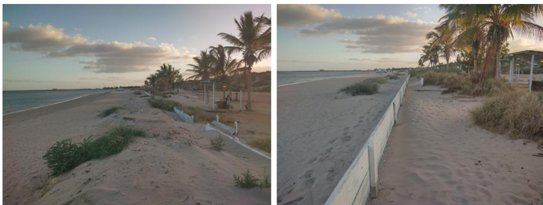
(a) Baffle fencing with constructed dune
