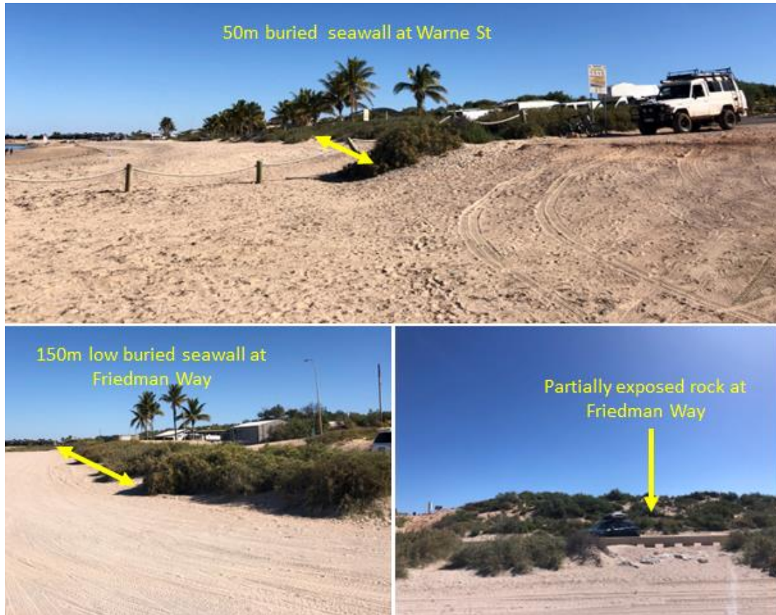
Figure 2-9: Partly Buried Seawalls at Warne St and Friedman Way
