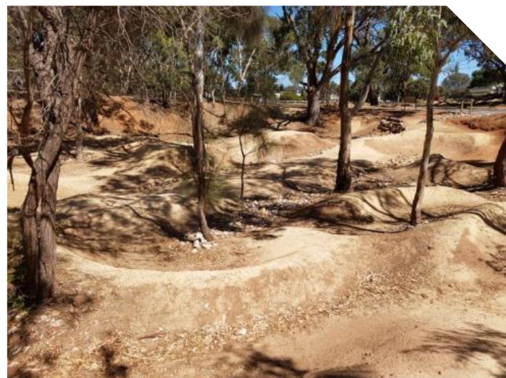
Image: 11 The Bowl Pump Track SA compacted gravel
