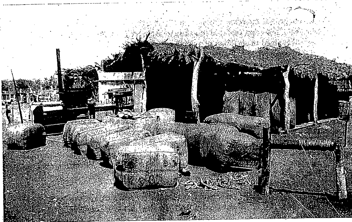
Photograph 3: Original shearing shed at Bullara Station
