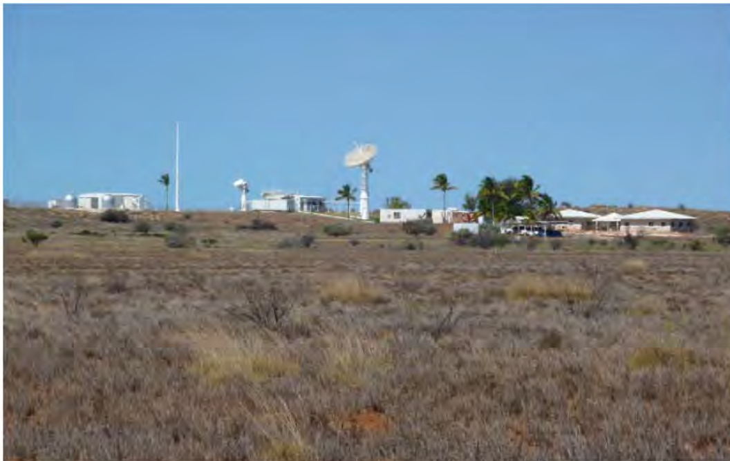
Learmonth Solar Observatory
