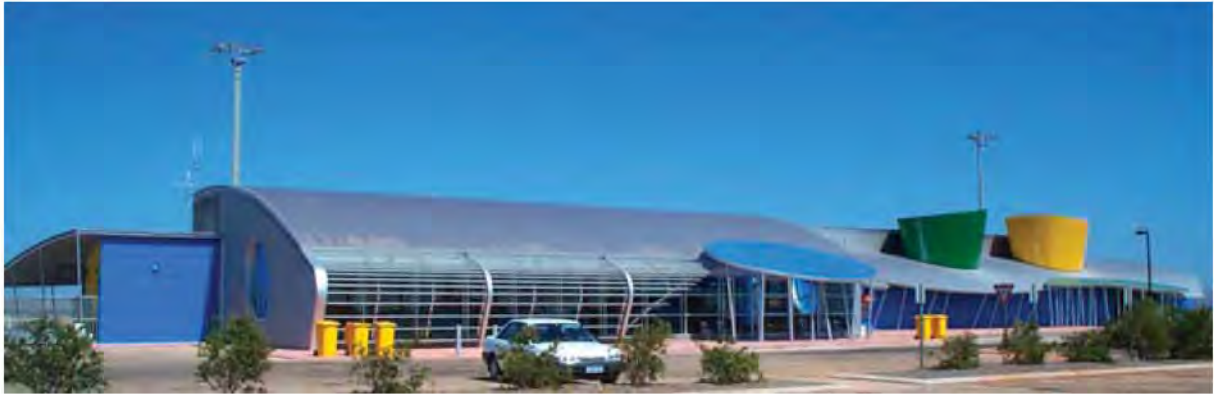
Learmonth Airport terminal
