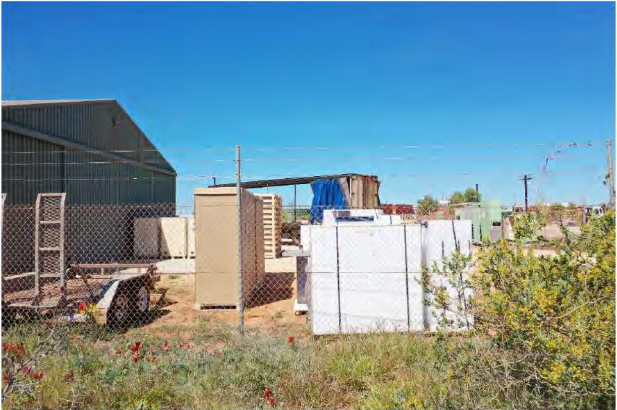
Figure 19: View of the equipment and material stored immediately adjacent to the proposed facility, and other equipment located on the frontage of the suite. Source: Ventia 2021
