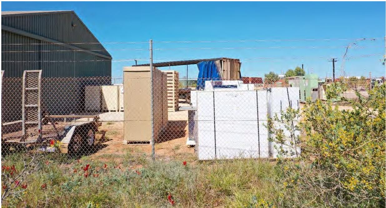
Figure 10 View east of proposed facility Source: Ventia 2021
