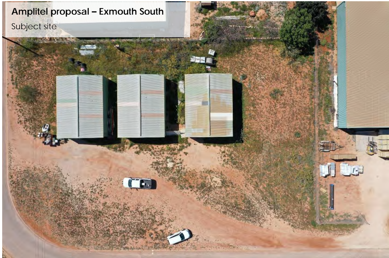
Figure 7: Subject site for Amplitel proposal – 14 Koolinda Way, Exmouth Source: Department of Planning, Lands and Heritage
