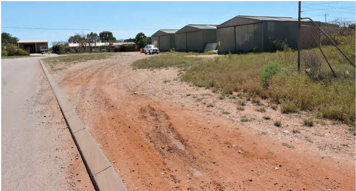
Figure 14 Existing access to subject site Source: Ventia 2021
