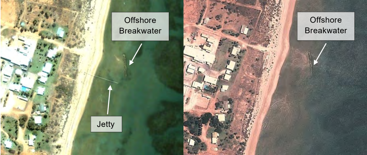
Figure 1.3 Site Coastal Structures in 2006 (left) and 2011 (right)
