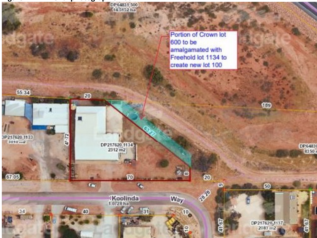
Figure 1: Aerial photograph of lot
