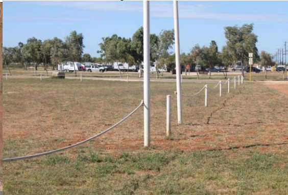
Photo 3 Example of Antenna Wire Fence
