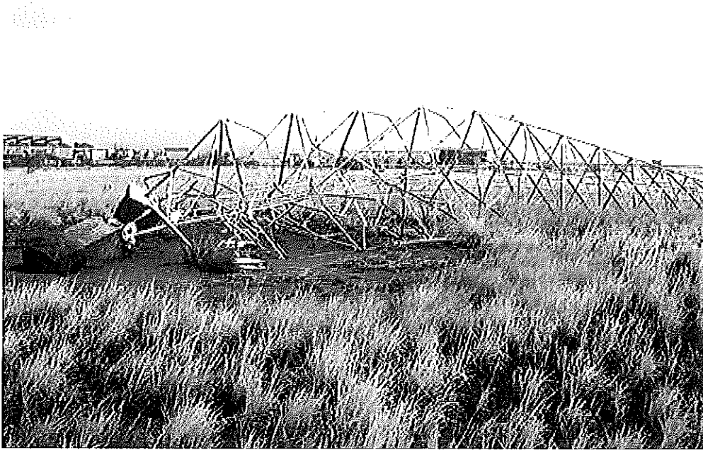
Fig. 17. Damage to communications mast near Learmonth. Photo courtesy of Matt Gould.
