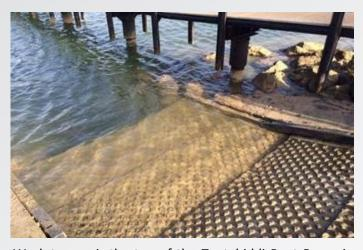
Work to repair the toe of the Tantabiddi Boat Ramp is scheduled from February 9-11. The boat ramp end panels have dislodged and sunk. While plastic kerbing is currently supporting and maintaining the alignment of the boat ramp panels, the ramps need to be repaired to prevent any further damage that would make the ramp unsafe.
