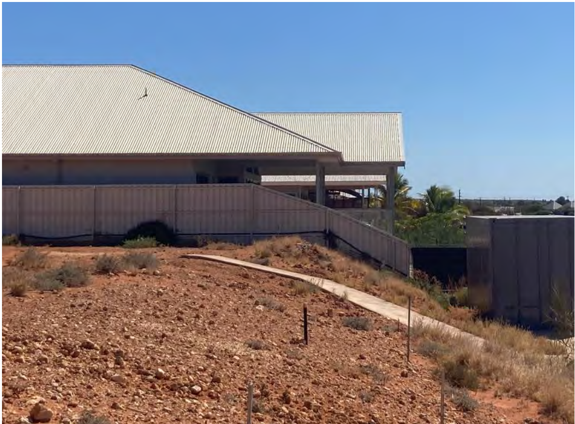
CDA area looking west
