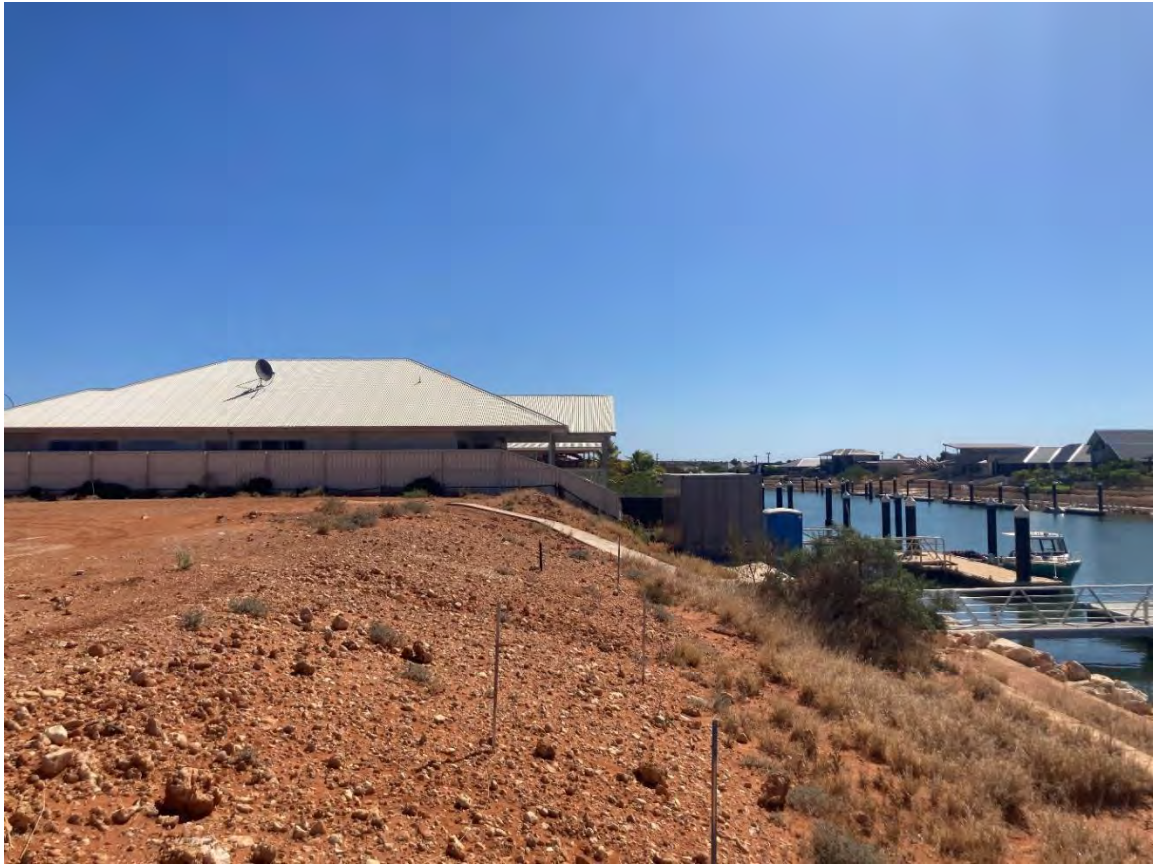
CDA area looking west
