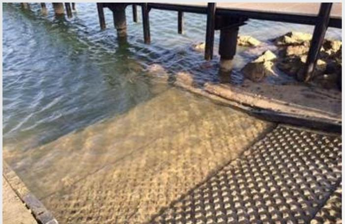
Work to repair the toe of the Tantabiddi Boat Ramp is scheduled from February 9-11. The boat ramp end panels have dislodged and sunk. While plastic kerbing is currently supporting and maintaining the alignment of the boat ramp panels, the ramps need to be repaired to prevent any further damage that would make the ramp unsafe.
