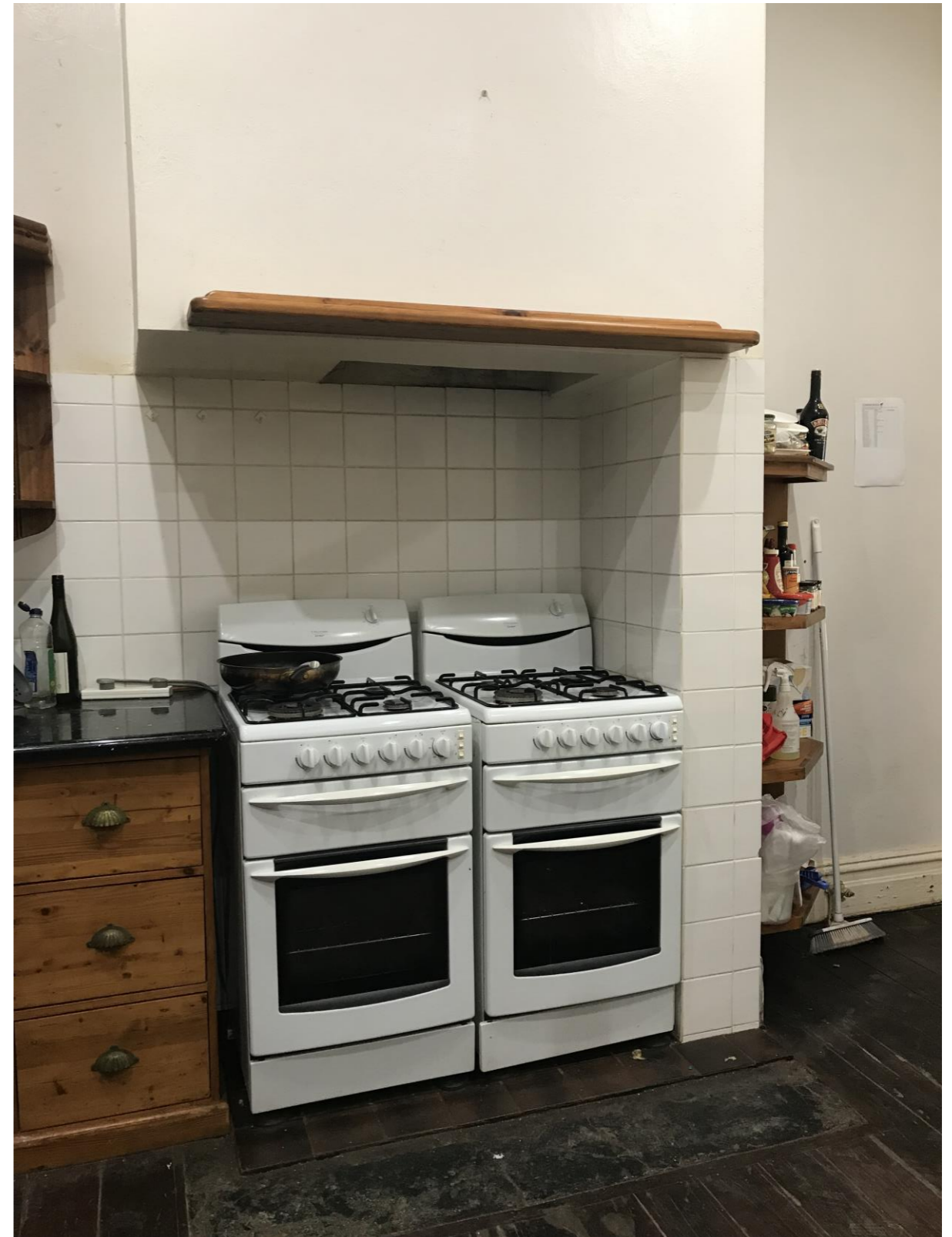
Photograph 9 Fireplaces to original living spaces have been modified to provide kitchen facilities (pictured) and robes. The remnants of the removed walls and hearth remain in the floor. Kerry Hill Architects, September 2019
