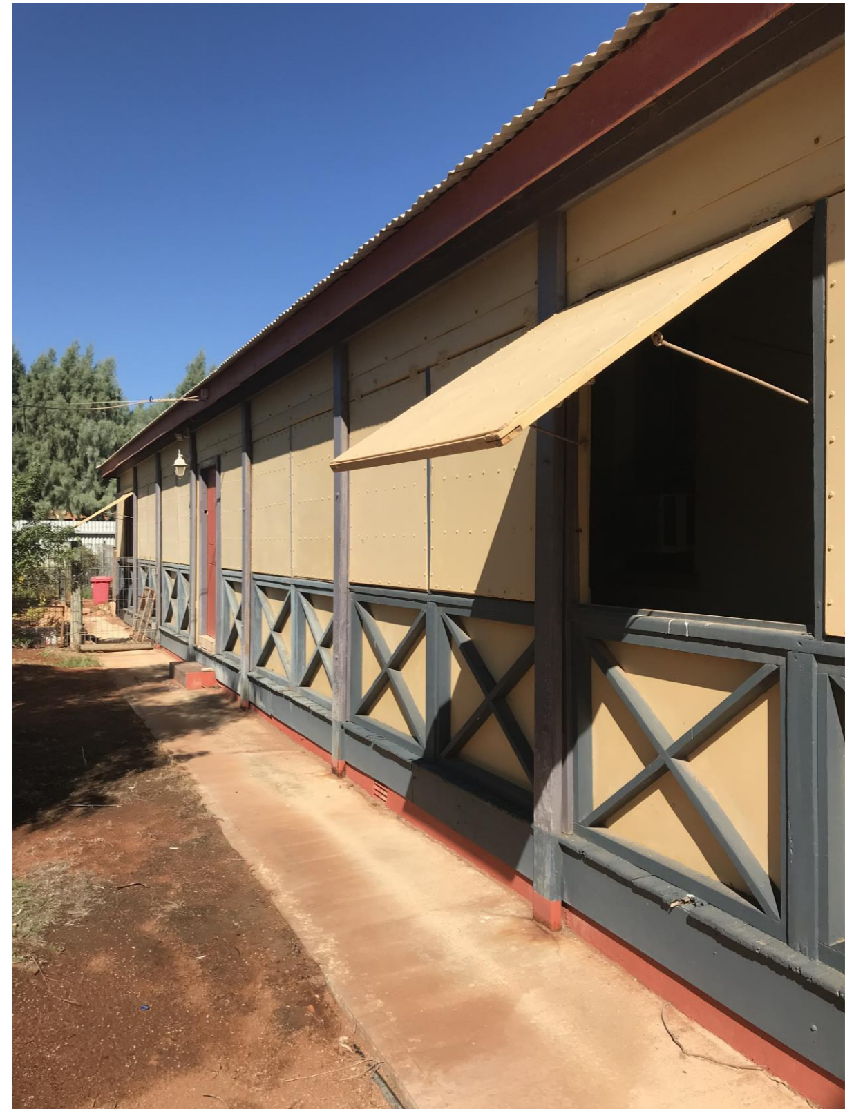
Photograph 3 East elevation. Kerry Hill Architects, September 2019
