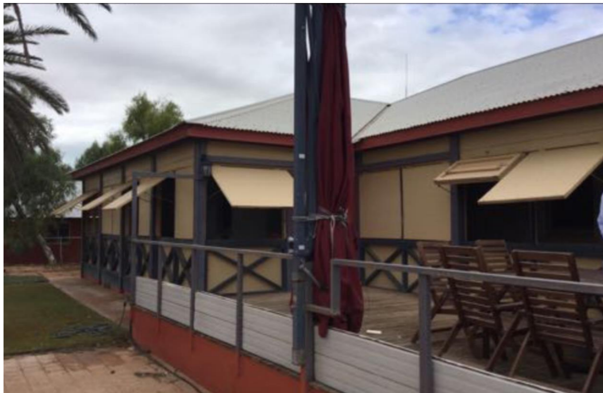
Photograph 1 North Elevation with central deck. BCWA report, September 2016
