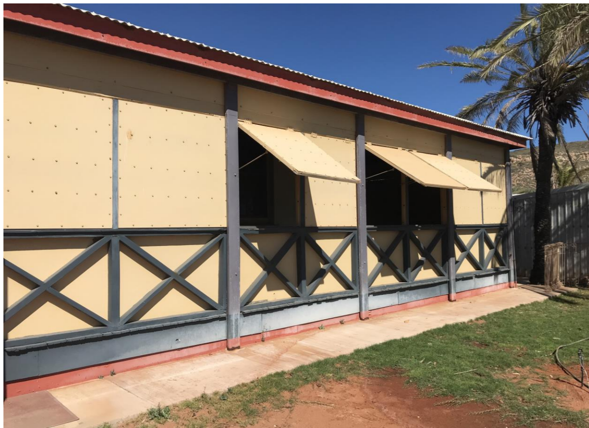
Photograph 2 West elevation. Kerry Hill Architects, September 2019
