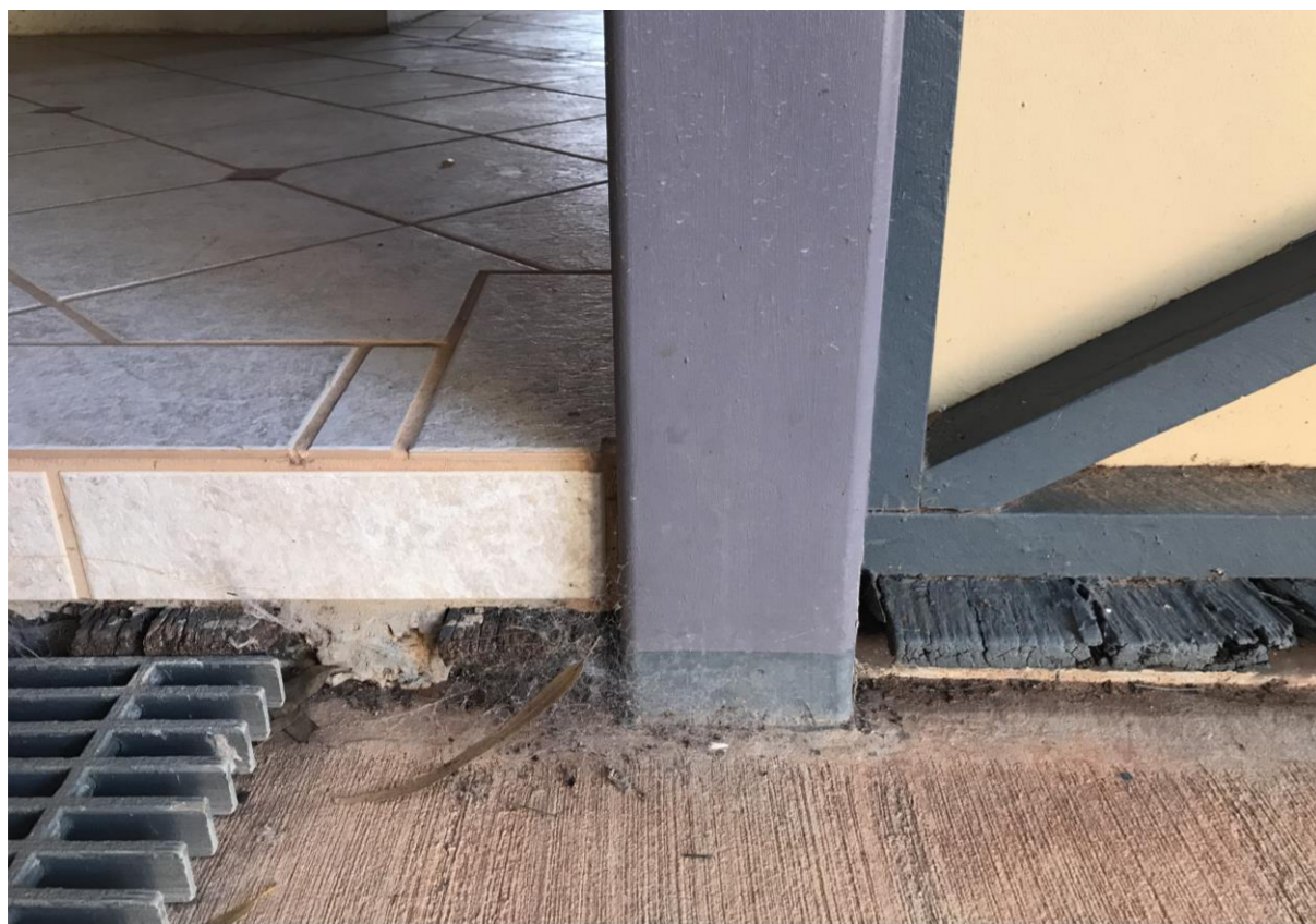
Photograph 7 Detail of concrete screed on verandah timbers. Kerry Hill Architects, September 2019
