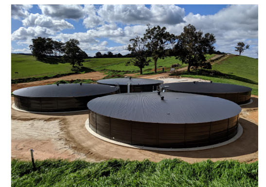
Picture of 2,000kL total water storage comprising 4 x 500kL tanks measuring 18.4m diameter x 2.31m wall height.
