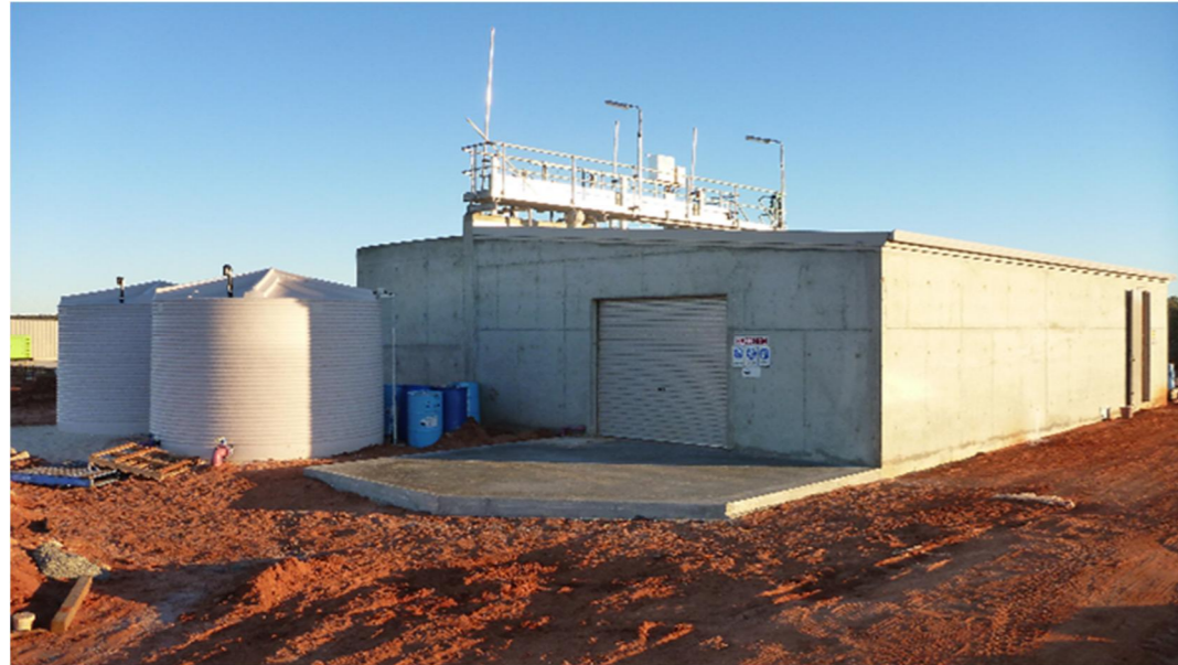
Figure 1 – Monkey Mia Dolphin Resort MBR wastewater treatment plant (2013)
