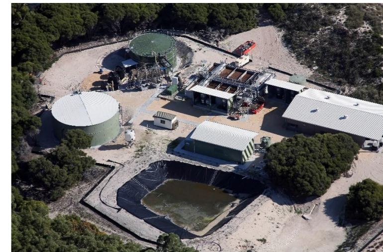
Figure 3 – Rottnest Island MBR recycled water plant
