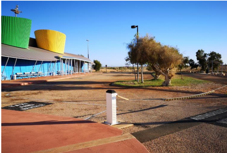
Figure 11 Existing arrivals bus loop
